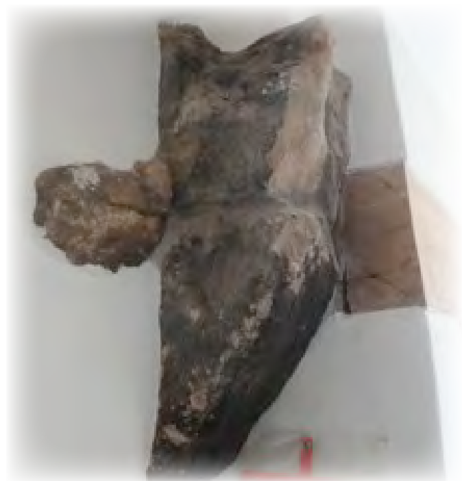
Left corbel with broken shoulder stone above and remains of lamp bracket on the left.
